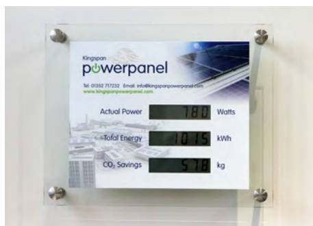
This display panel in Reception gives instant information about how much energy is being generated by the photovoltaic panels on the roof.
