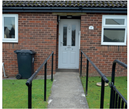
Above: Grab-rails fitted
